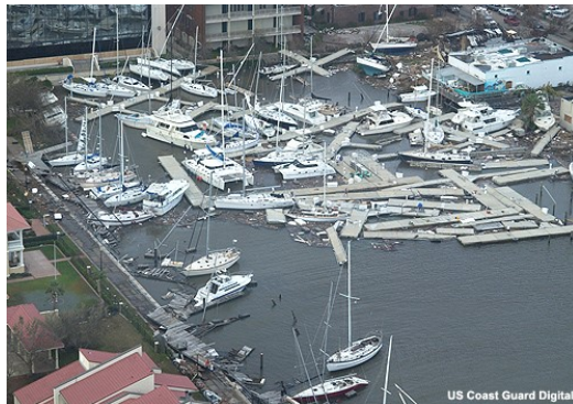
(b) Damaged Boats in a Marina
