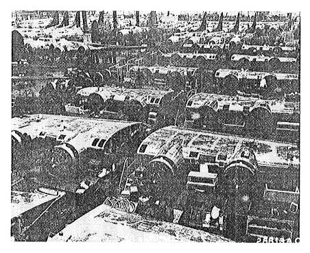
Fig. 4.4 B-17Es in Plant No. 2: inboard wing subassembly *Source:* USAF Museum (Wright-Patterson AF Base).
