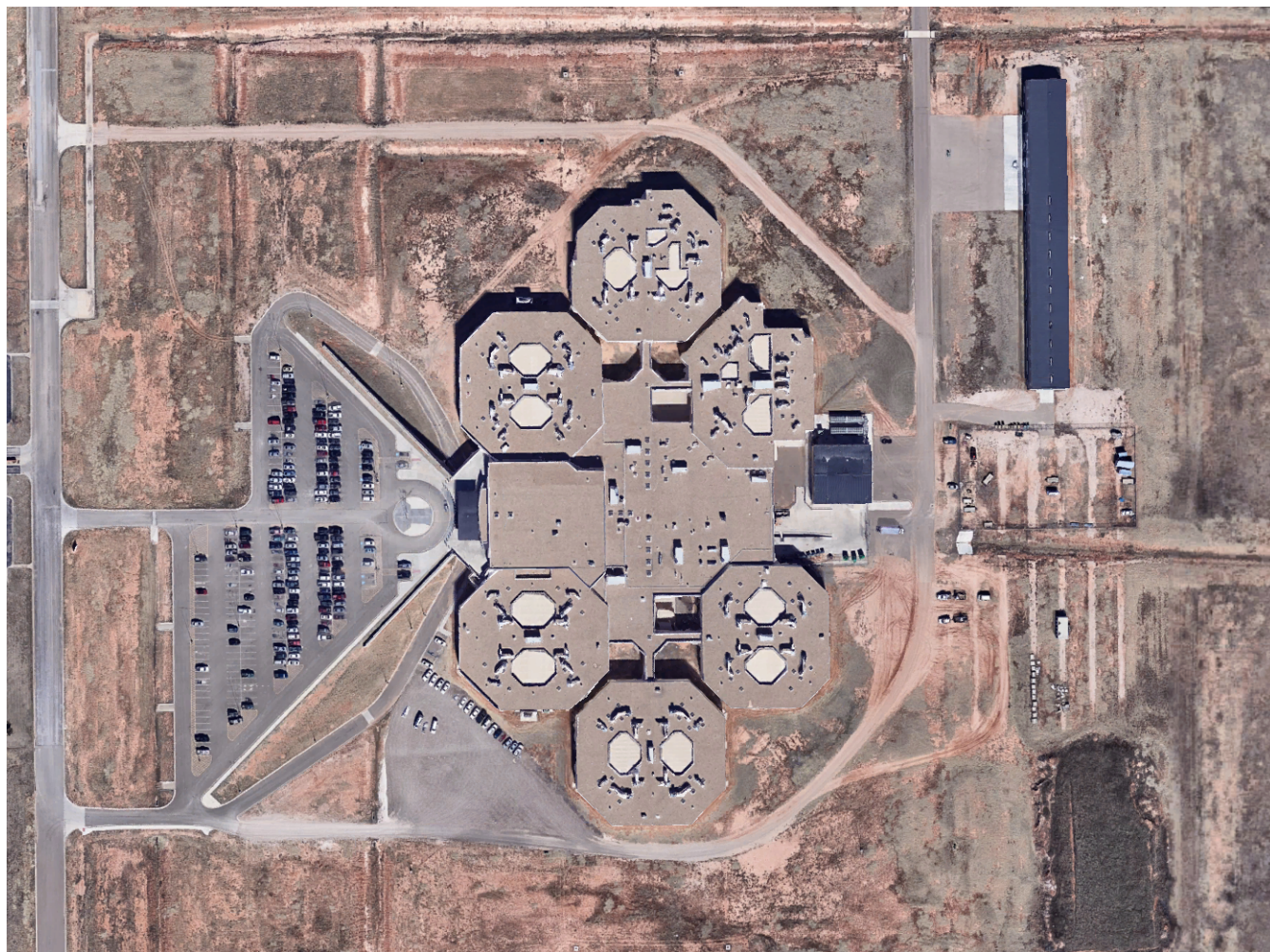
Figure B.1: Aerial View of the LCDC
