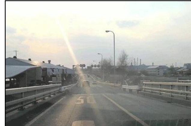
Miyagi prefectural road, Route 240
