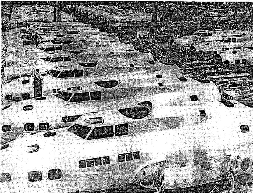
**Fig. 4.5** B-17Es in Plant No. 2: forward fuselage subassembly
